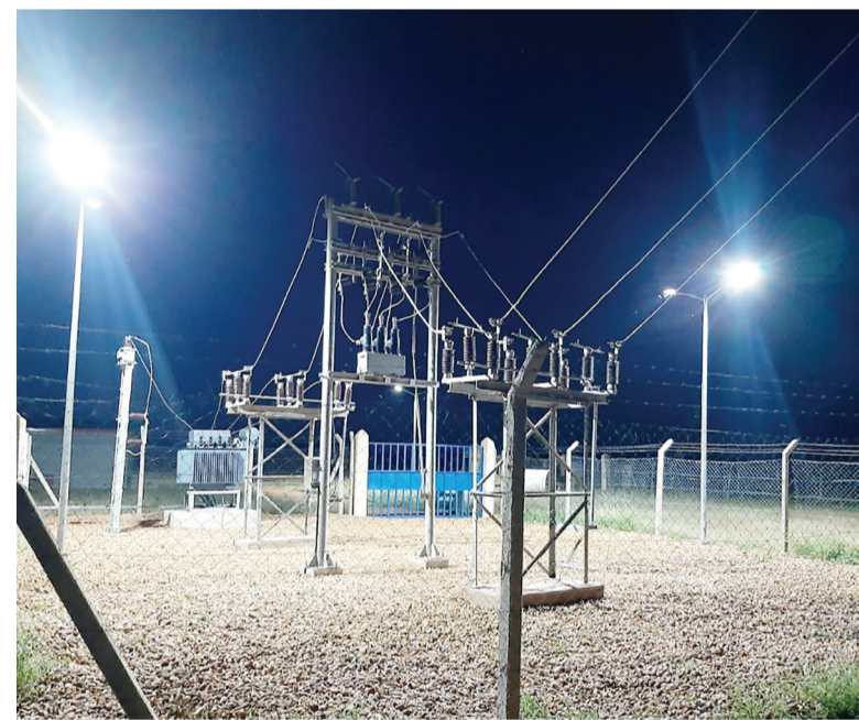
Solar mini-grid evacuation substation in Buna, Wajir County.
