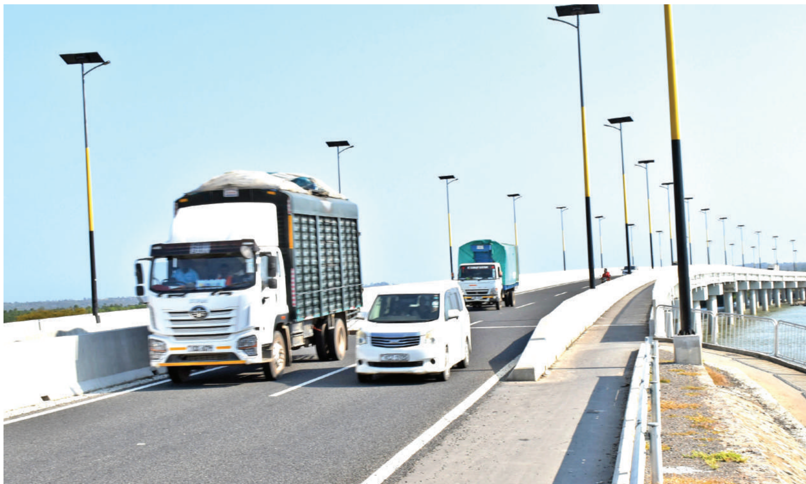
Motorists use the newly constructed Dongo Kundu Bypass in Mombasa County.
